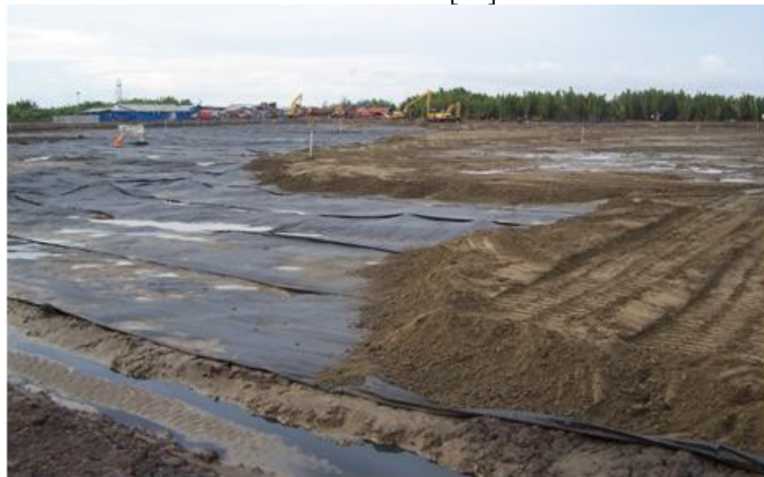
Fig. 9 The use of geo-textile for separation between foundation soils and the backfill material [48]
