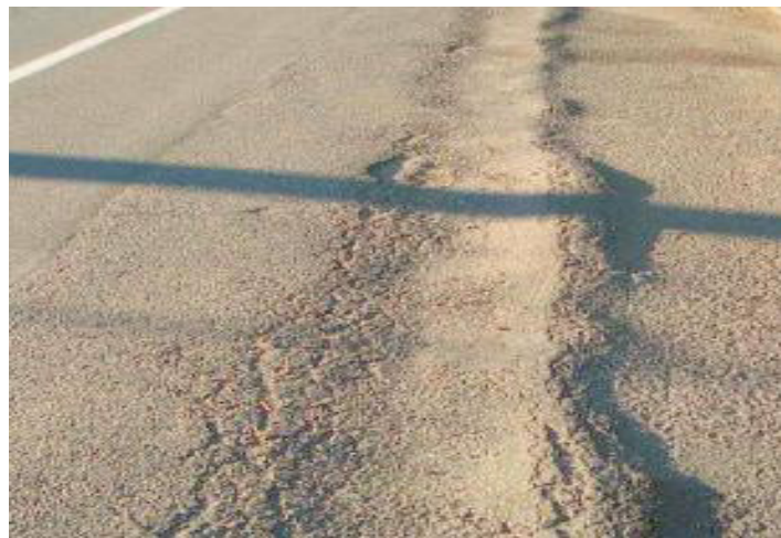
Fig. 6 Rutting in Flexible pavement [14]
